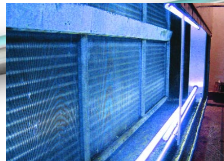
Stainless steel construction, ready for inhospitable HVAC environments.
