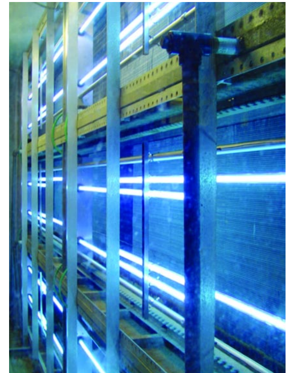
The Ultravation UVMatrix™ SI-Series utilizes our patented T3 UVC lamp system featuring Philips UV lamps—the lowest environmental impact UV lamps manufactured today. The T3™ system emits up to 40% more germicidal UV using low cost and low power-consuming standard configuration UV lamps. The SI-Series' patented flexible design was created to accommodate any HVAC configuration for new or retrofit installations.
